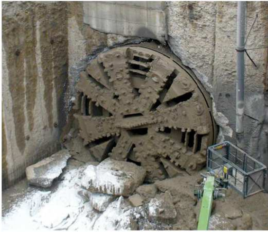
Above left: Breakthrough of an 8.16-m Wirth EPB TBM equipped with TunnelTec tools on the Castellanza metro project, Italy. The cutterhead is equipped with both static rippers and scrapers and disc cutters with carbide bullet inserts. Right: Disc cutters shown on the cutterhead of a 9.90m-diameter NFM Technologies TBM on completion of 1140m in a single month for the Madrid-Gijon high-speed railway route
